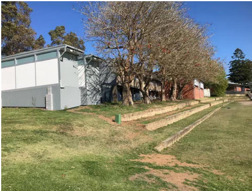
Photograph 4; Terracing and suspected filling surrounding buildings and retaining walls
